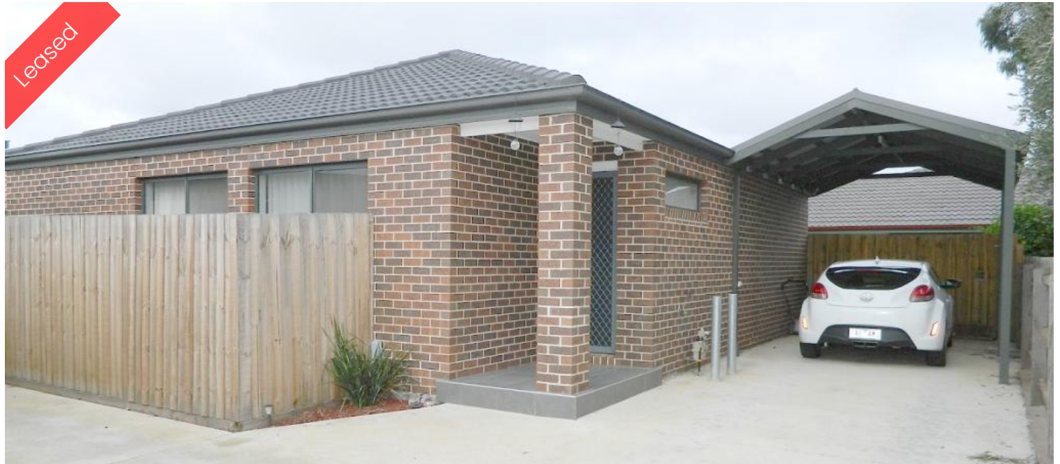
Unit 1, 39 Grace St, Melton South
