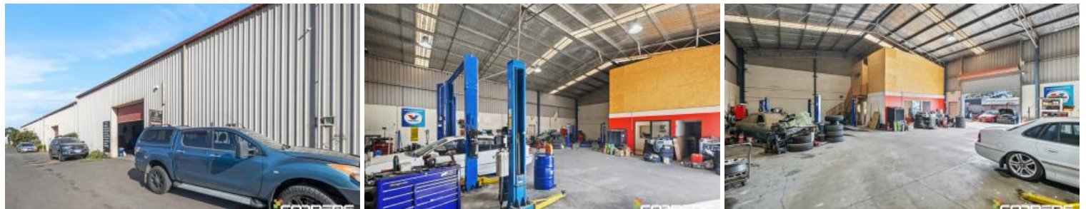
Factory 2, 21 Melton Valley Drive, Melton
