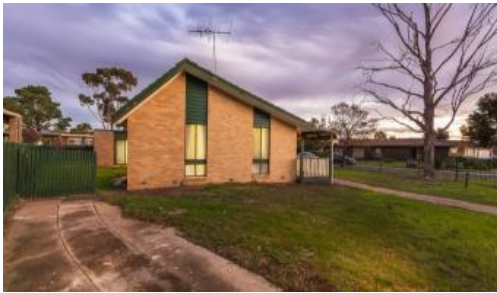
15 Linlithgow Way, Melton West
